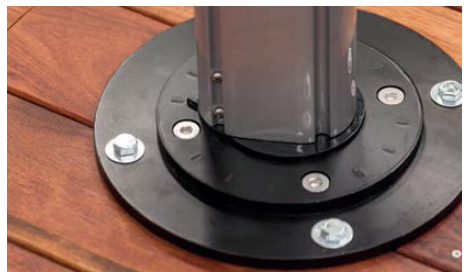
Figure C Align the indicator arrow with a notch
